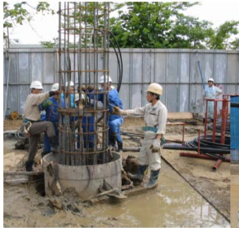
Lowering the reinforcement cage with U-tube loops
