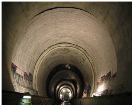
Energy tunnel/anchor systems (Brandl 2006)
