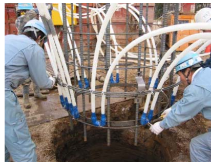
Reinforcement cage equipped with circulation loops
