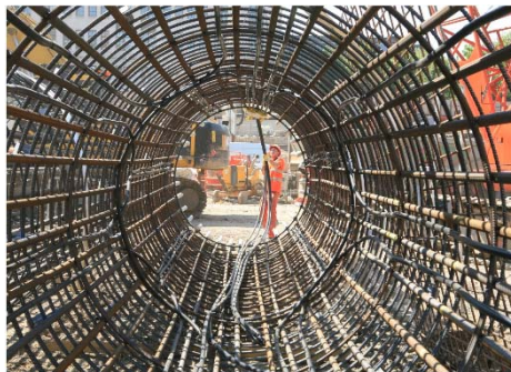
Reinforcement cage equipped with circulation loops
